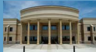
December 2006 Construction completed on Hall of Administration.
