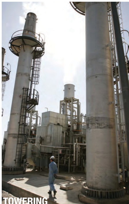
This Iranian heavy-water production facility could produce bomb-grade material.
